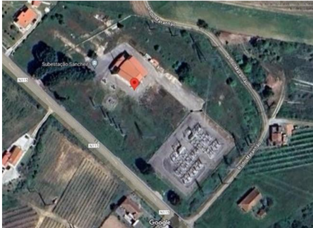
Figure: The primary substation of the OH MV line in Óbidos town in the district Leiria.
